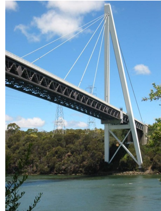
Batman Bridge Tas painted in an Ethyl Zinc Silicate remained corrosion free for 20 years. Only the A frame was topcoated and remained corrosion free for 30 years
