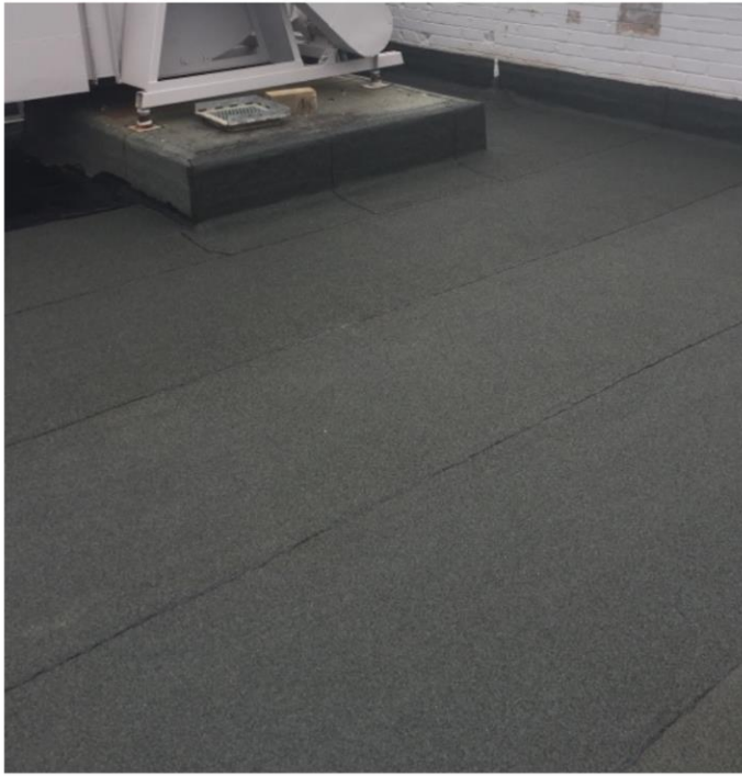
Roof: Torch-On System
